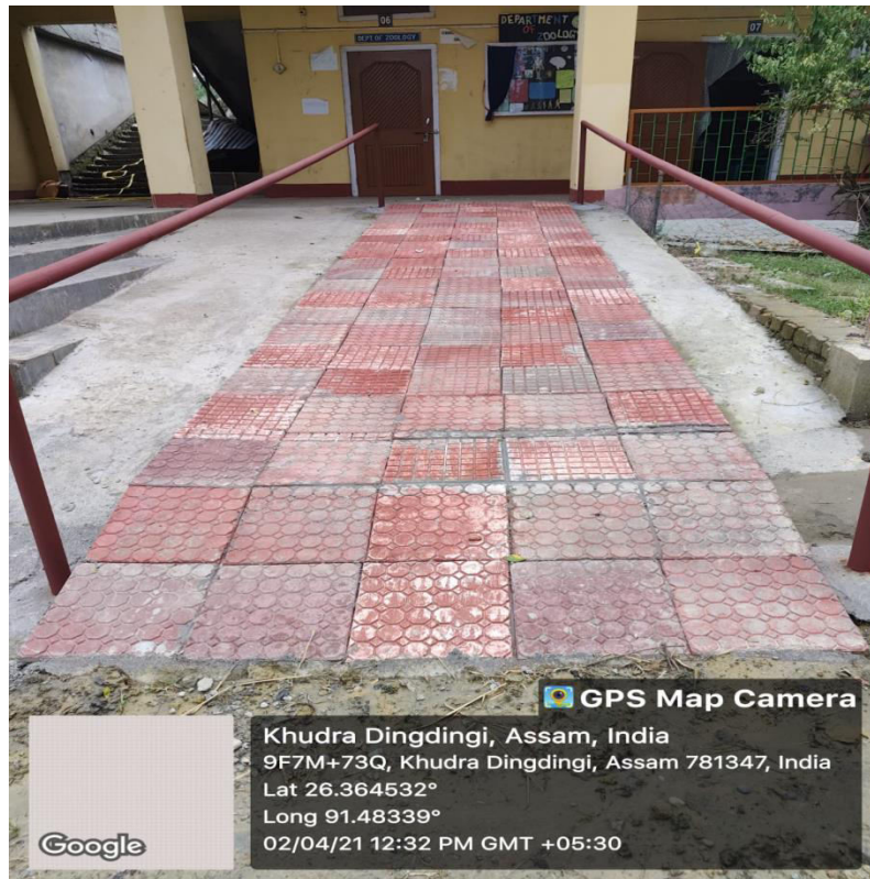
Photos of Ramp and Rails:
